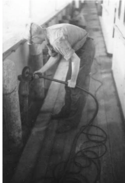
(11) Cadet Briggs Wire Brushing Stand Pipes After Chipping
